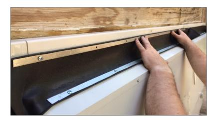
Fasten the Retainer Strip with screws to the flat face of the Top Rail just below its center screw. The ends of the Retainer should be placed at the middle of each Top Coupler.
