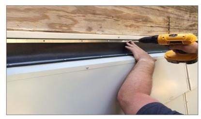
Next, fasten a screw though both overlapping seals to secure them to the Vertical Rails and also at each end rail. <a href="Update">Update</a>: Use Large Washer under screw head. Washer provided with hardware. <a href="Do Not over tighten causing damage to the seal">Do Not over tighten causing damage to the seal</a>.
