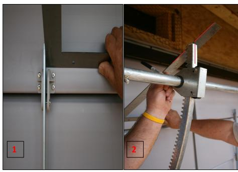
With all Shutter Units <u>hanging freely and in the exact</u> <u>same near closed position</u>, firmly tighten down both set screws with a 4mm Allen wrench while the Pinion is positioned on the marks. Continue this procedure for each Pinion.
