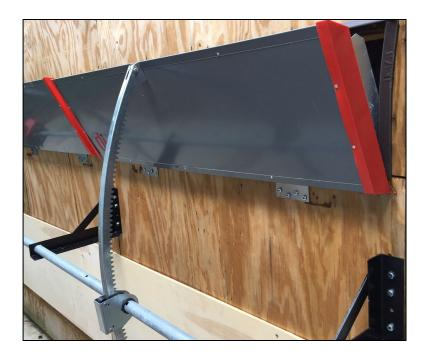
Our Torque Tube is available in 20' lengths with swaged ends to provide any required length. Install one each Torque Tube Hanger with each Vent.
